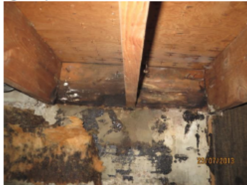
Perimeter with rigid fibreglass removed
